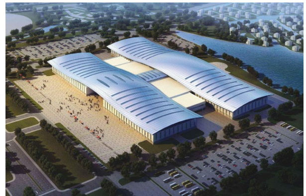
Aerial View of Tianjin Meijiang Convention Center
